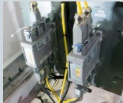
ethernet switches on board
